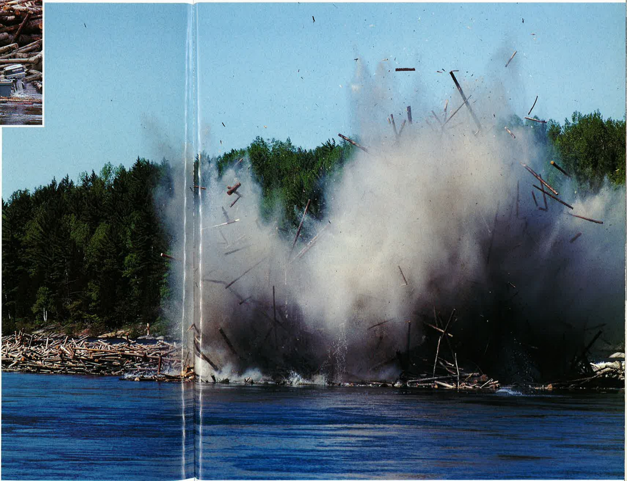
Carefully placed charges of dynamite provide a practical solution (above) to log jams that occur as the water level drops through the warm months. Small jams on rocks and sand bars can grow swiftly into enormously complex tangles of logs (above left).
